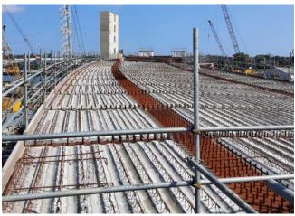
With the OmniaPlanks complete, the teams stayed on the Southern Approach, continuing with the installation of the reinforced steel bars, in preparation for the concrete pours. These 10 pours were done in a specific order, to enable proper curing of each section.
