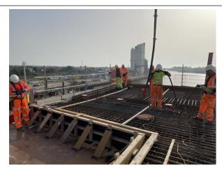
In addition to the deck pours, due to the weight of the opening section of the bridge being on the Southern side, a special "encapsulation pour" took place in early September over the end of Pier 4. As the description says, the concrete encapsulates the end of the steel work over the pier, binding it and the steel structure together allowing extra support and strength.
