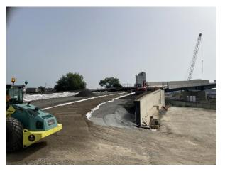
At present we are at the asphalt stage of the road network, both on the roadways and the new footpaths. Once these are completed road markings and street furniture/signs will be installed.
