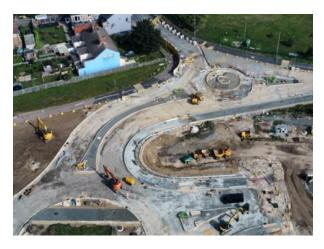
The new larger roundabout starts the incline up the Northern Approach and over the bridge. The approach itself comprises of 2 retaining walls which is filled with compacted aggregate before the layer of asphalt is installed.
