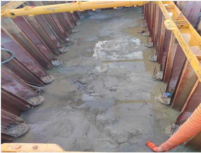
A – Pier 4 Piles Cut and Cleared Out
