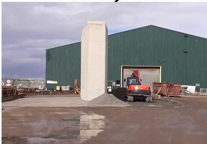
C – Pier 6 Completed and Backfilled
