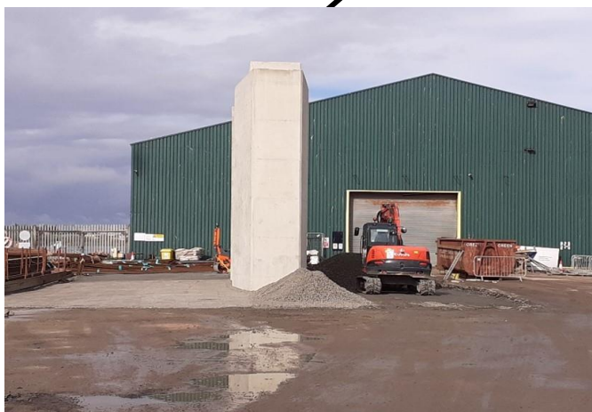
C – Pier 6 Completed and Backfilled
