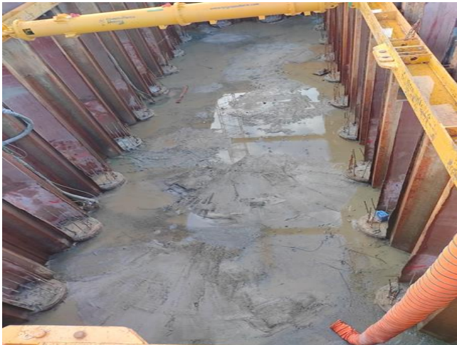
A – Pier 4 Piles Cut and Cleared Out
