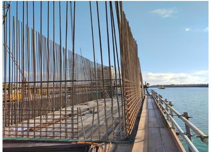
B – Pier 5 Formwork for Stem
