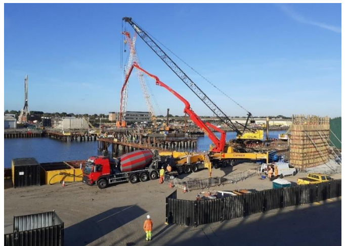
B – Cofferdam 5 - Preparing Wet Plug
