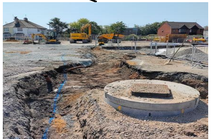
D – Southern Roundabout Works
