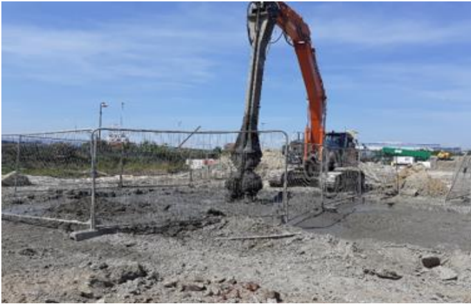
A - North Approach – Deep Soil Mixing
