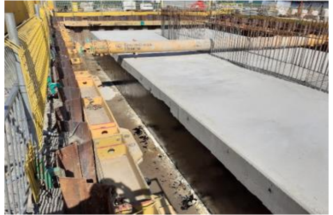
B – Pier 6 Pile Cap
