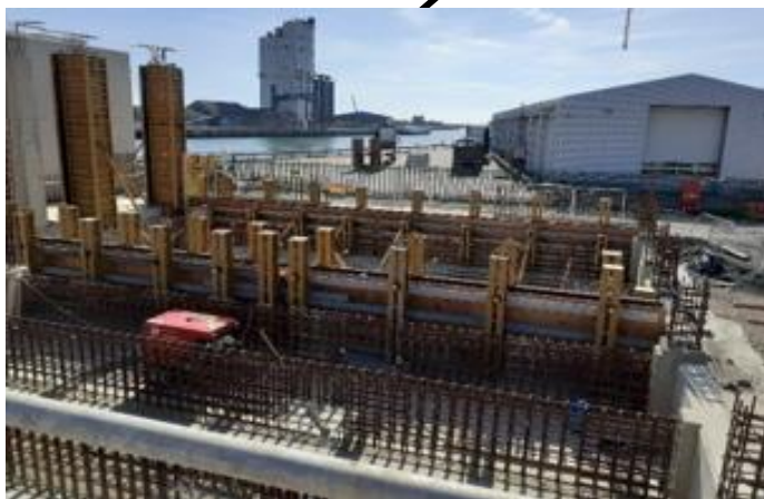
C – Control Tower Plant Room
