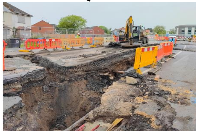
D – Southern Roundabout Works
