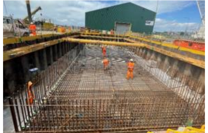
B – Pile Cap 6 – Reinforcing steel
