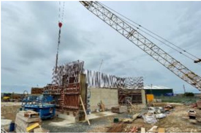
A - North Abutment – Wall E Shutters
