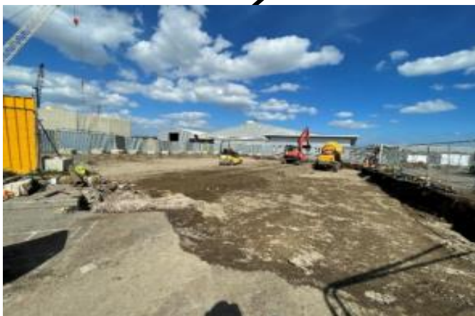
C – Pier 1 – Laying Piling Platform
