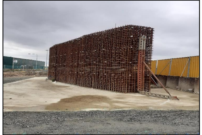
B - Pier 7 – Reinforcing steel
