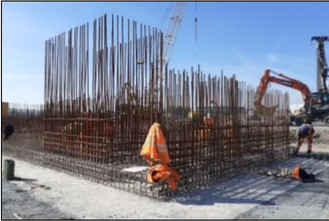
A - North Abutment Reinforcement
