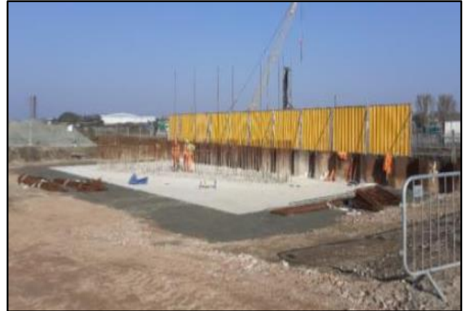
B - Pier 7 – Pile Cap Backfilled
