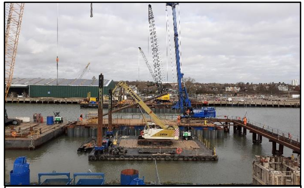
B - Pier 4 – Rotary Bored Piling
