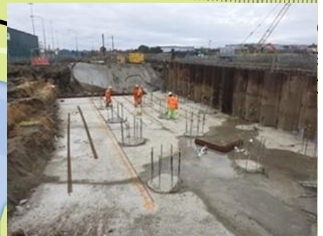
Pier 7 –Pile Cropping
