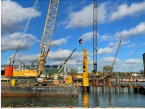
Pier 4 – Bearing Piles Testing
