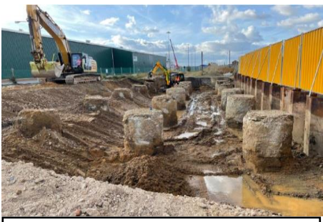
Pier 7 – Pilecap Excavation
