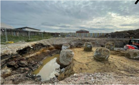
Pier 2 – Pilecap Excavation
