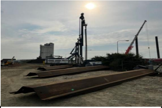
Network Rail – Sheet Piling Installed
