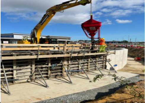
Lings Wall – Concrete Pouring
