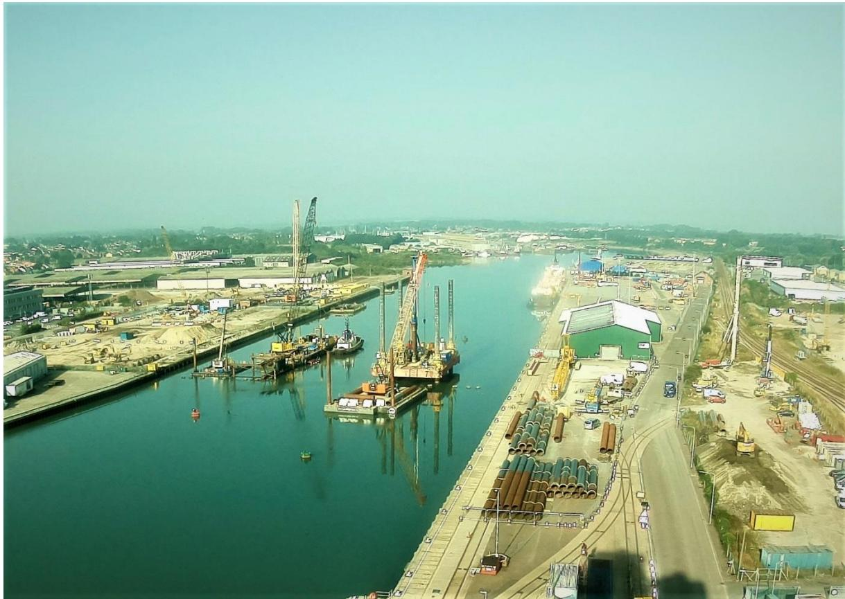
After a long period of planning and preparation, the first marine construction works started on 10<sup>th</sup> August when the first pile was installed into Lake Lothing. A pile is a cylinder type foundation inserted into the ground to support heavy loads.
