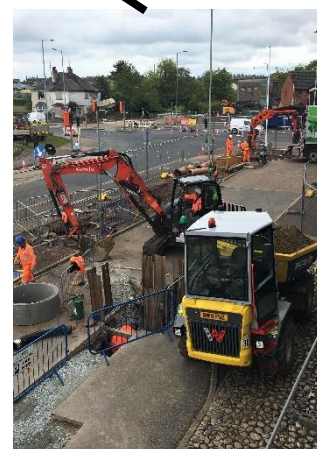
Riverside Rd Sewer Installation
