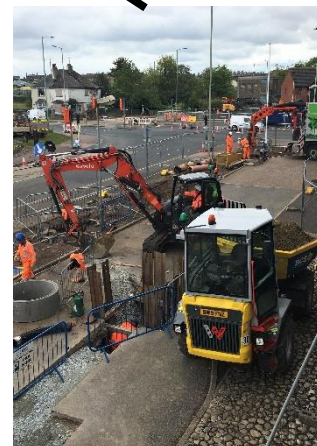
Riverside Rd Sewer Installation
