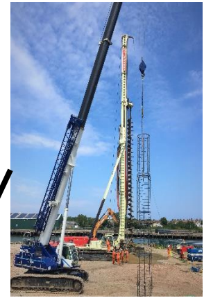
Piling Works – Pier 3
