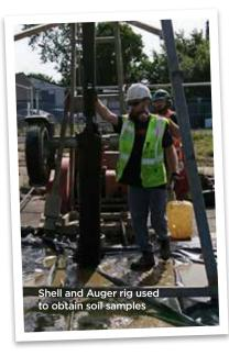
The works include digging trial holes and deep boreholes both on land and in the water. The findings will help finalise the detailed design for the new bridge piers and foundations.
